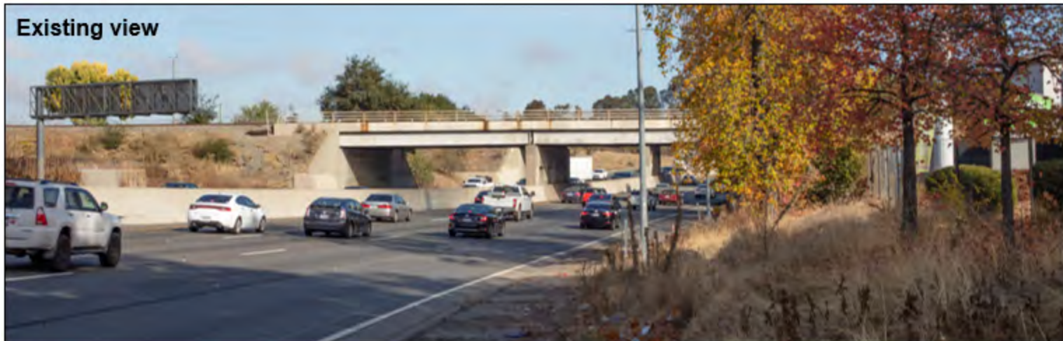
Figure 3.1-4. Key Viewpoint #2a – Existing and Simulated View of B Street Railroad Bridge Crossing (view looking north from eastbound shoulder of Capital City Freeway)
